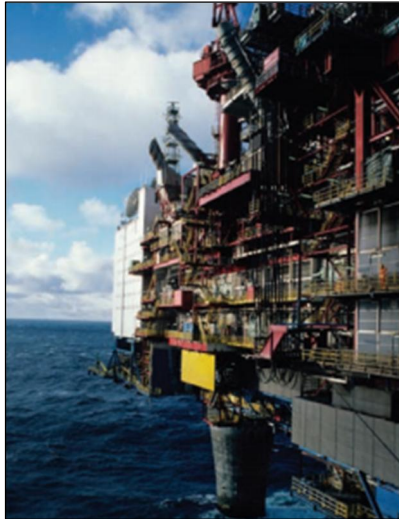
Figure 1: Natural Gas and Oil Processing Platform
