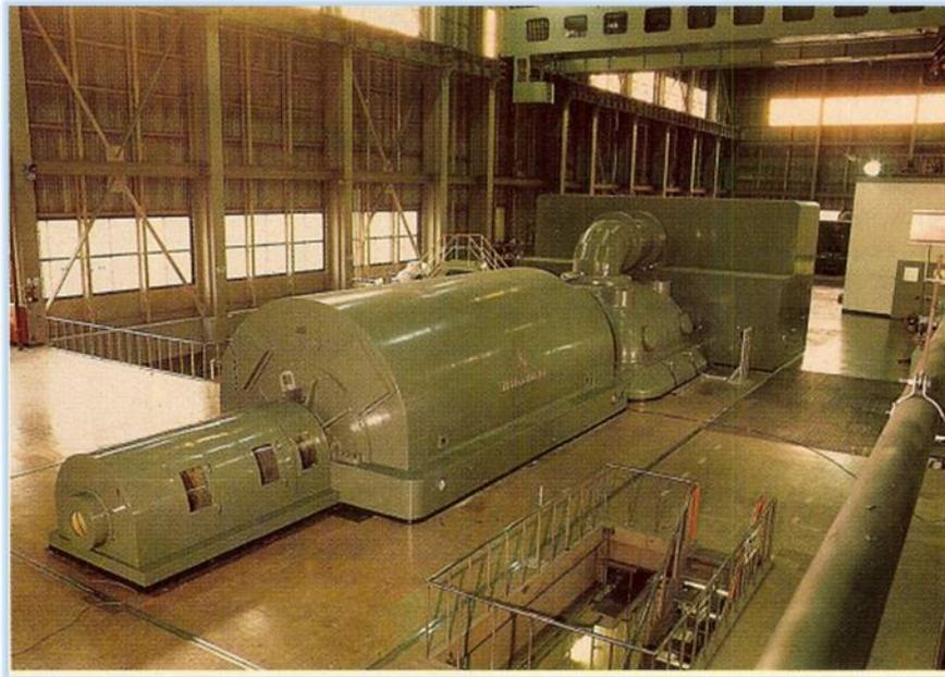
*Figure 1: A steam Turbine Generator, ca. 1985. The largest component is the generator, which would be about 10 to 15 feet high. Behind the generator is the low-pressure turbine.<sup>1</sup>*
